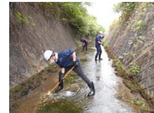
Clean up of the Oku-Osugidani River
