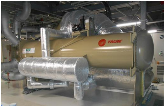
Centrifugal chiller with Non-Freon refrigerant
